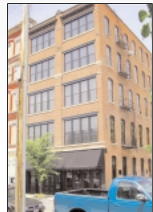
Electronic Ark office building
